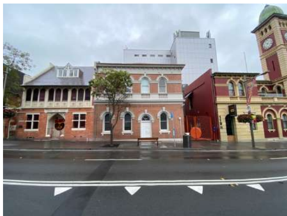
Figure 6: Photo taken from Redfern Street showing the original 1913 telephone exchange building in the centre, the neighbouring St Vincents Church building to the left and the Redfern Post Office building on the right.
